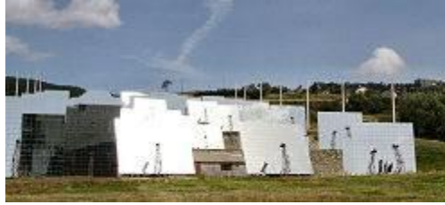
Fig: The array of mirrors is controlled by a computer and turn with the sun.
