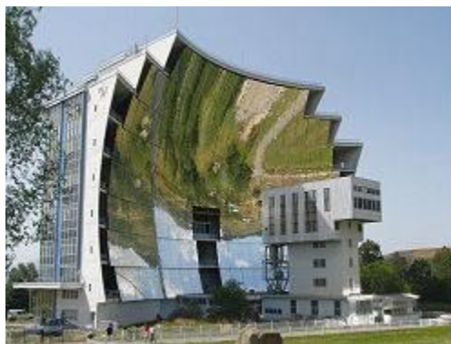
Fig: The Solar Furnace of Odeillo; the parabolic shape of the giant solar collector is evident here.
